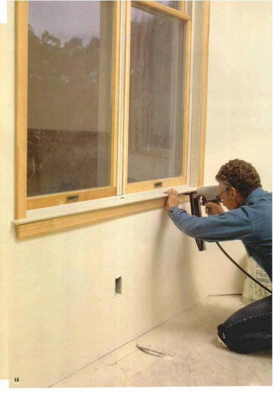
backing here because the screwed connection between the jamb extensions keeps them from being driven out of alignment.
